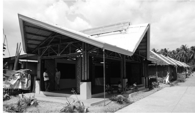
Figure 3: Estudio Damgo (ED) 2 Multipurpose Hall completed 2014. (Credit: Foundation University.)
